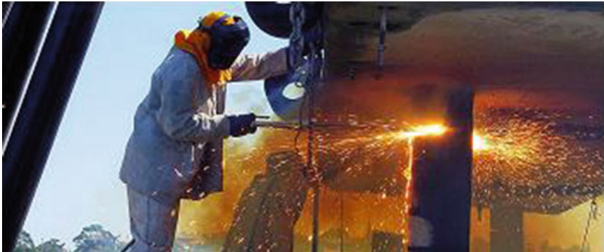
Fig. 2.4 Cutting of reinforcement through high temperature (Prakash 2014)
