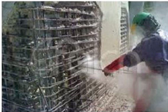
Fig. 2.5 Demolition by water jet (Prakash 2014)
