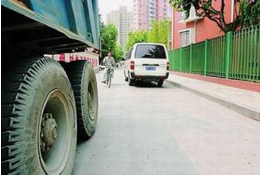
Fig. 1.3 RAC pavement in Shanghai, China (Li 2009). This pavement was designed for a width of 7 m and 240 mm height. 50% RCA was used. The RCA was derived from the highway of an airport
