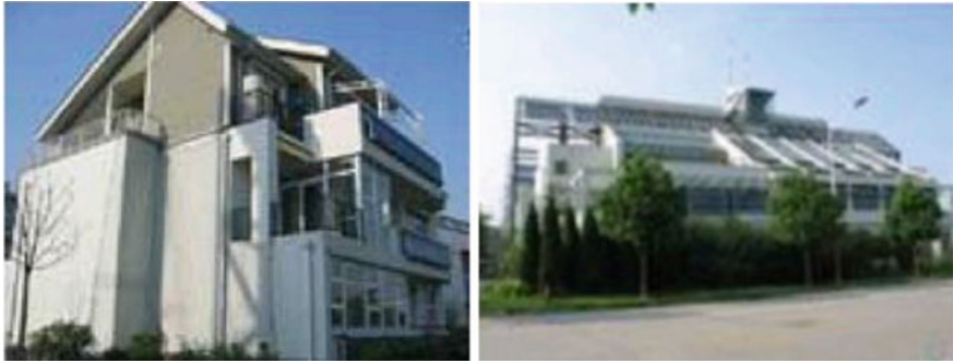
Fig. 1.4 Shanghai ecological building, China (Li 2008). This was a demonstrative ecological green building constructed in Xinzhuang, Shanghai, in 2004 with a total area of 1900 m 2 . Large amount of RAC (388 m 3 ) was used mainly in foundations and walls. The RCA was produced by crushing old concrete pavements and structural elements
