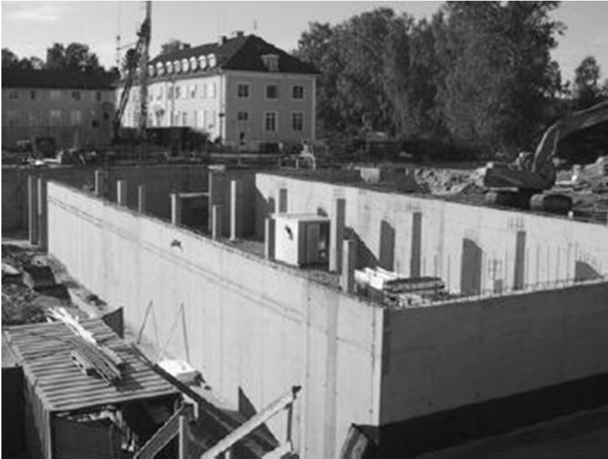
Fig. 1.8 New high school building in Norway (Mehus and Hauck 2002), in which 35% recycled coarse aggregates were used in foundations, basement walls, and columns
