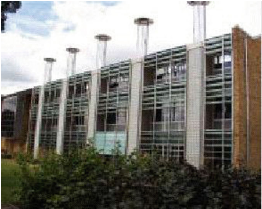
Fig. 1.5 The BRE office building in Watford, UK, 1995/96 (BRE 1998). For the foundations, a C25 mix (75 mm slump) was used with a minimum OPC-based cement content of 350 kg/m 3 and a maximum free water–cement ratio of 0.50 was required. For floor slabs, a C35 mix, also with 75 mm slump was specified. Over 1500 m 3 of RAC supplied for foundations, floor slabs, structural columns, and waffle floors
